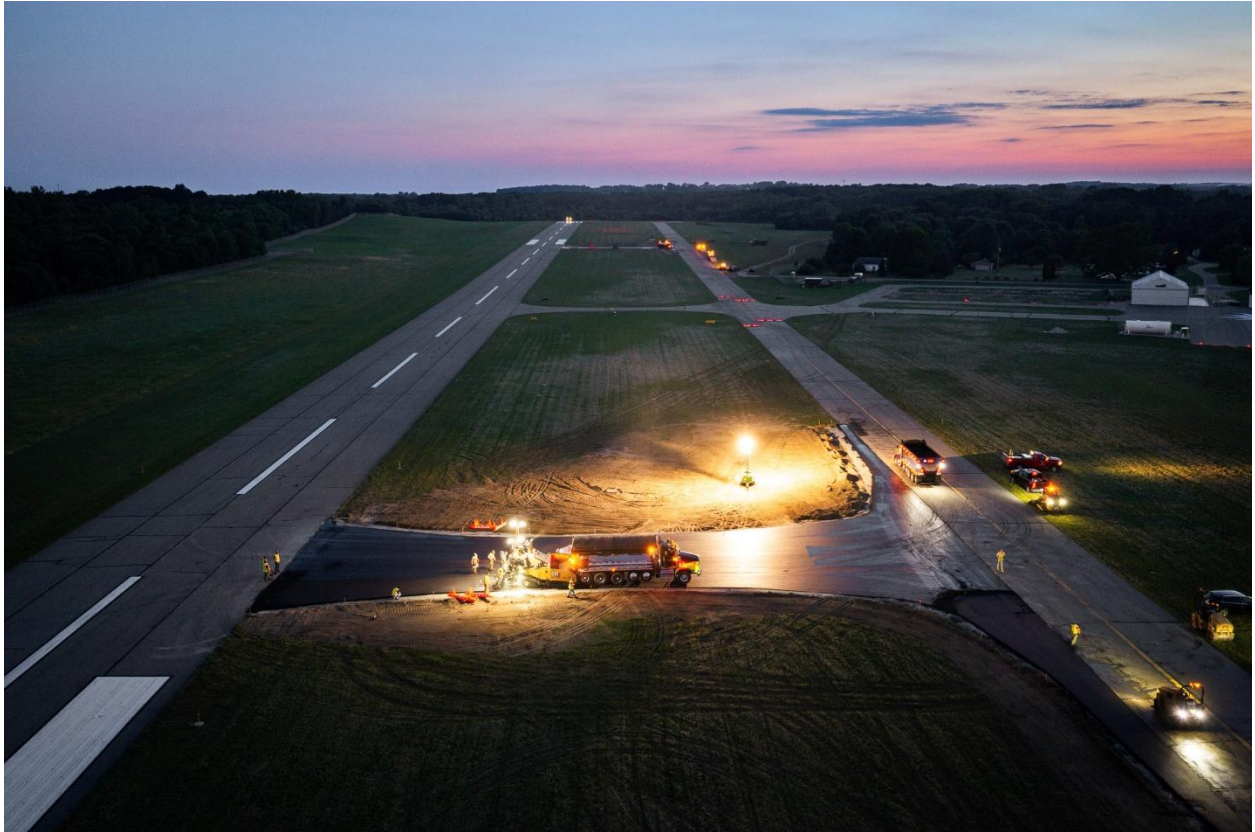
New east side taxiway connector
