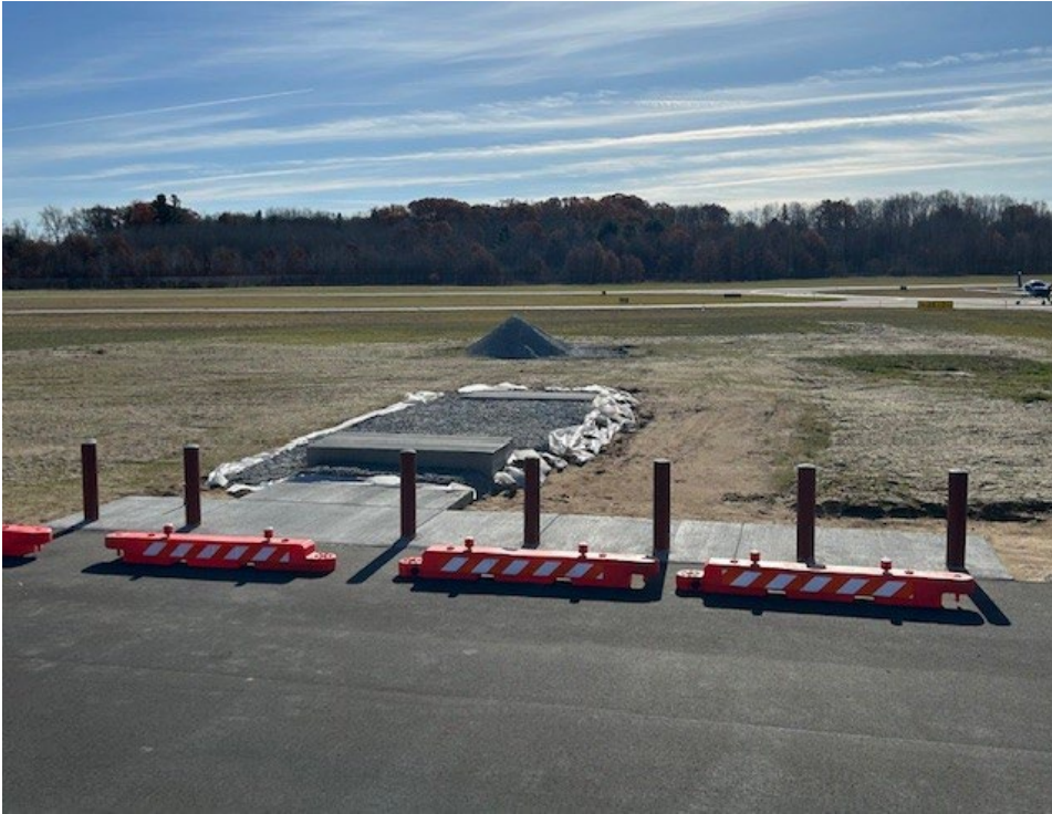
Jet Fuel Farm Crash Protection (these will be covered with safety yellow bollard covers)
