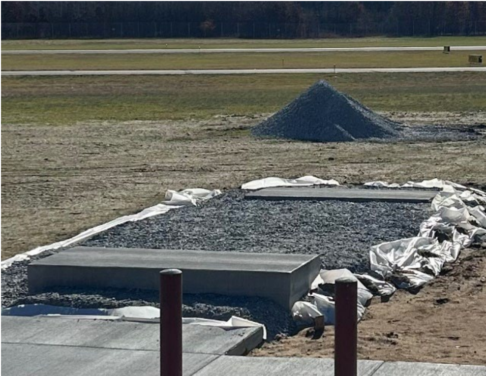
Jet Fuel Farm tank footings
